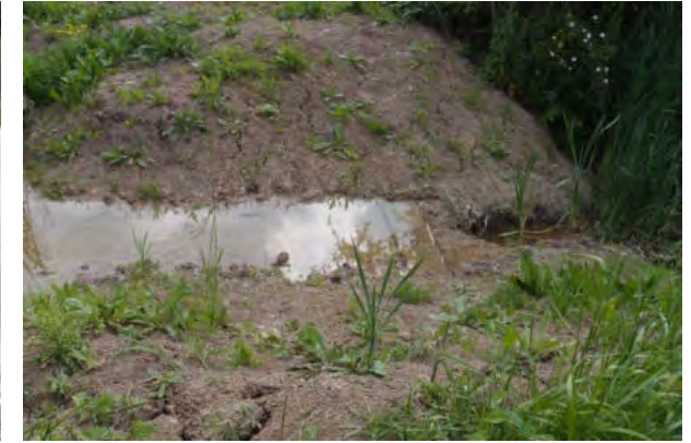
Photograph 30 Ditch outfall from New Pond.
