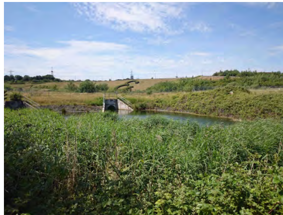
Looking upstream towards discharge from balancing pond
